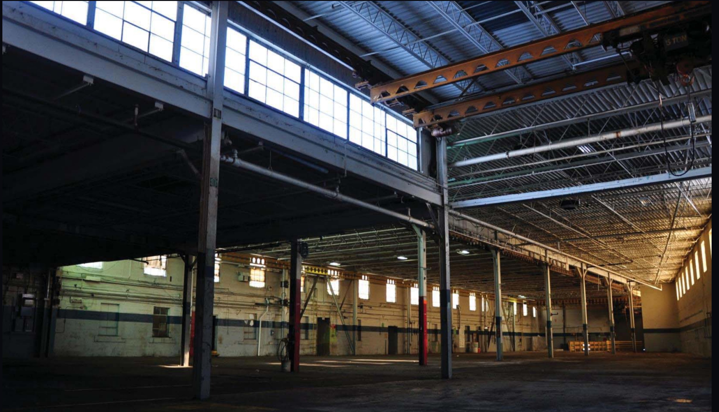
INTERIOR OF EXISTING STRUCTURE 08.31.2015
