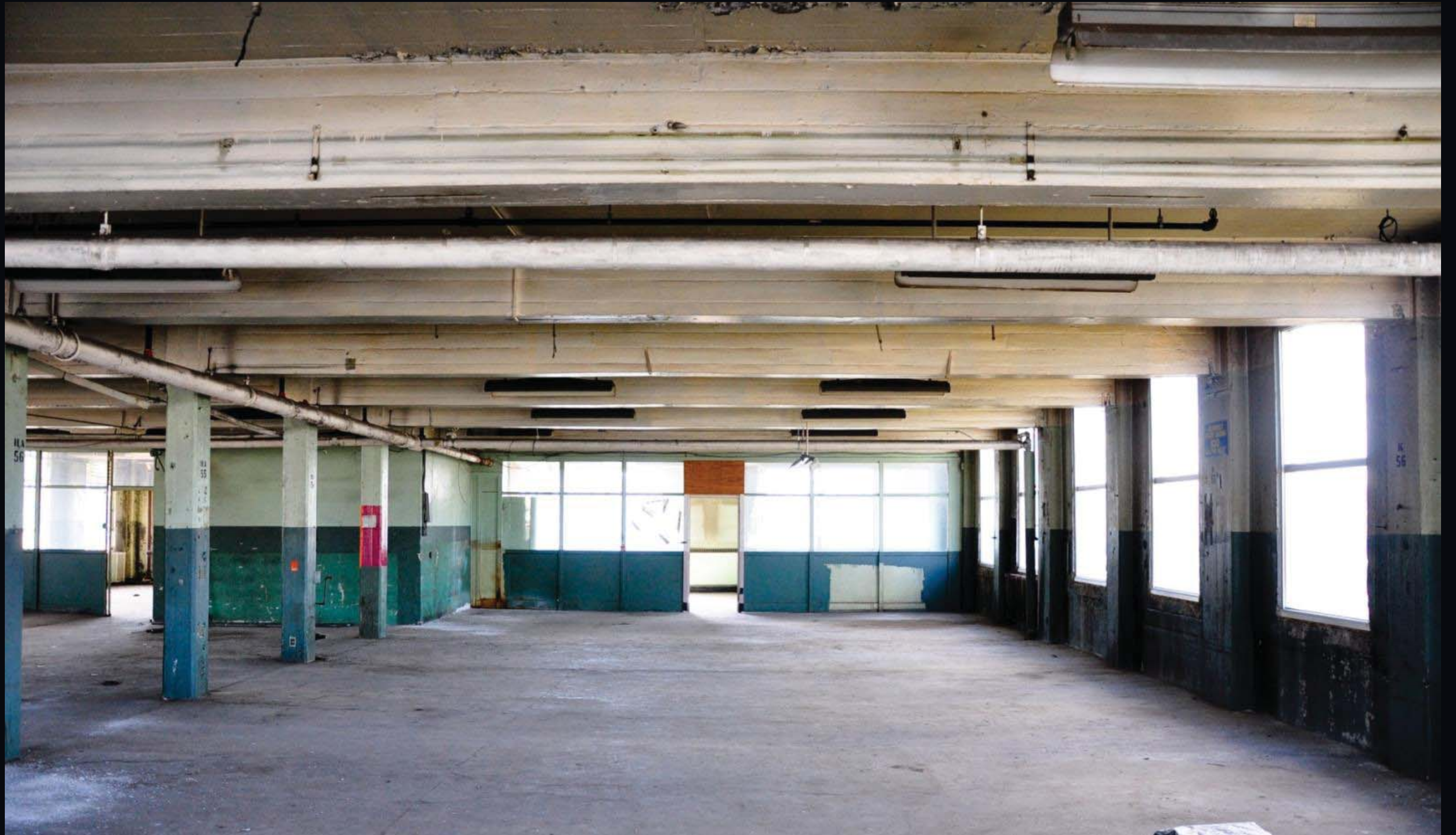
INTERIOR OF EXISTING STRUCTURE 08.31.2015
